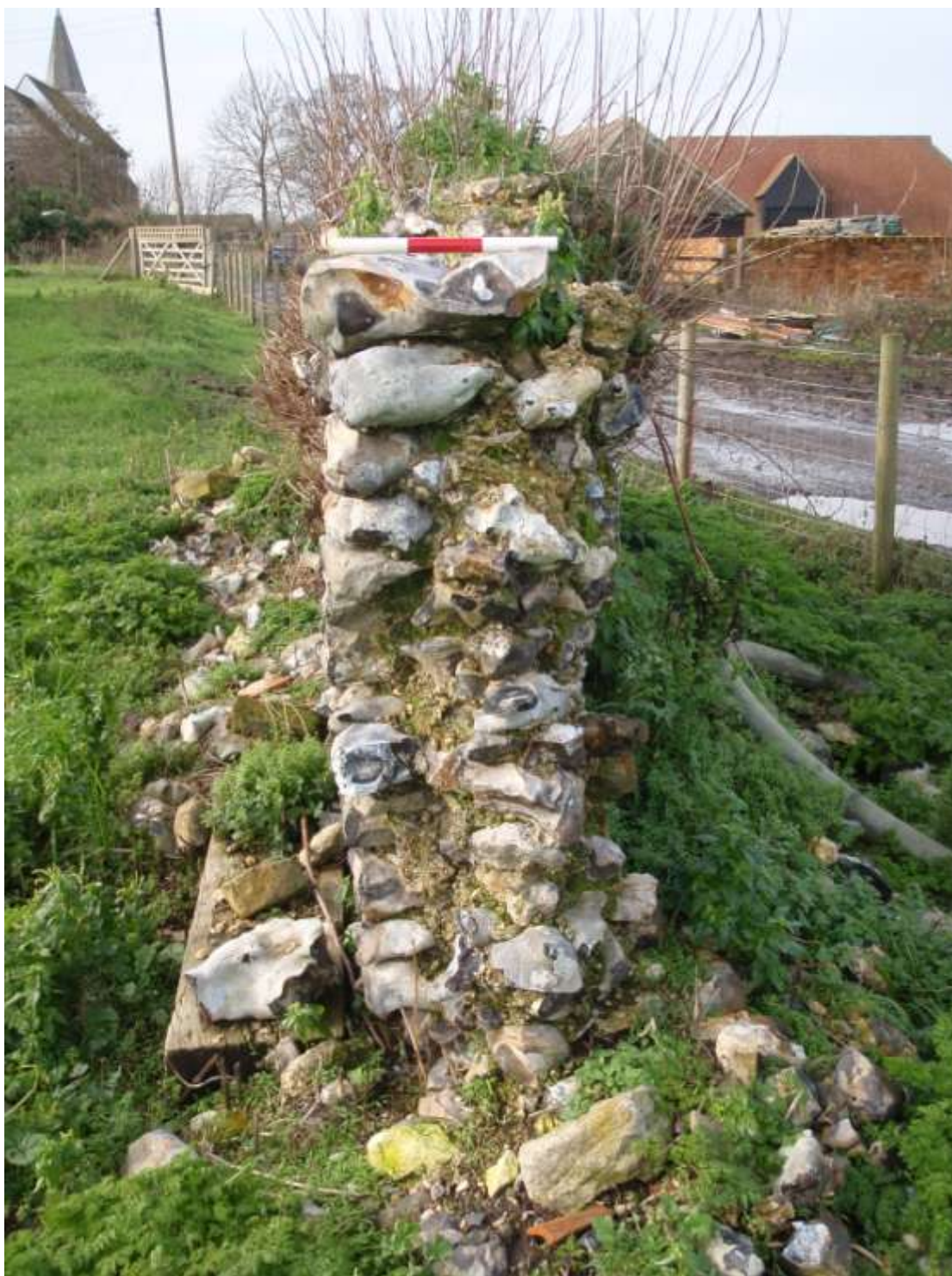
Plate 7. General view of upstanding medieval wall (looking west)
